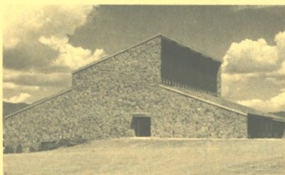
COMBINED administration and library building, Nazarene Bible College.
