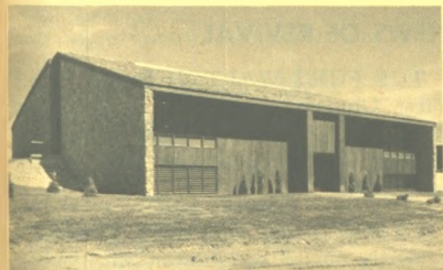
NEW classroom building, Nazarene Bible College.
