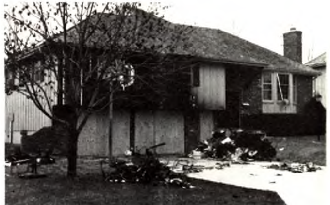
The parsonage of the St. Paul's Church of the Nazarene in Kansas City, Mo., was destroyed by fire March 13. The fire started in the garage as Pastor D. L. Huffman and his family were preparing for bed. Everyone escaped safely, but the house and two cars in the garage were declared a total loss. The home and its contents were insured.
